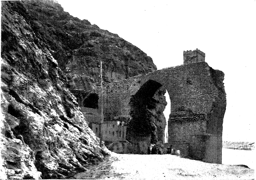
58. PIERS AND ARCH OF PUL-I-DUKHTAR BRIDGE, ON LEFT BANK OF KĀSHGĀN RIVER
